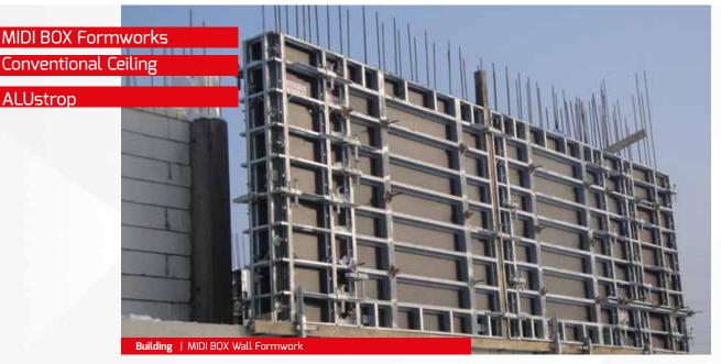
MIDI BOX formwork systems are spatial components used for multiple installations. They are intended for forming strip foundations, walls and square or rectangular posts, horseheads, elevator shafts and atypical structural components, among other things, in virtually every facility.
