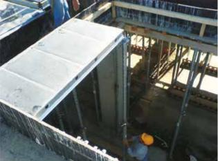
In general, the ALUstrop system makes the installer/carpenter work very easy as it is repeatable and the complexity of its installation is very low. However, it is not the cheapest formwork solution, the time saved during its installation provides an added value when considering this system as a whole.
