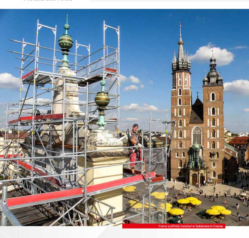
ALTRAD-MOSTOSTAL manufactures steel and aluminium frame Mostostal Plus scaffolds. The system consists of basic components such as: frames, rails, braces, platforms, toe boards and jacks.
