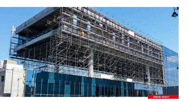
The scaffold load-bearing capacity depends on its width and length of platforms used to install the specified assembly and may range from 2 up to 6 kN/m2 (loading classes as per PN-EN 12811-1:2004).
