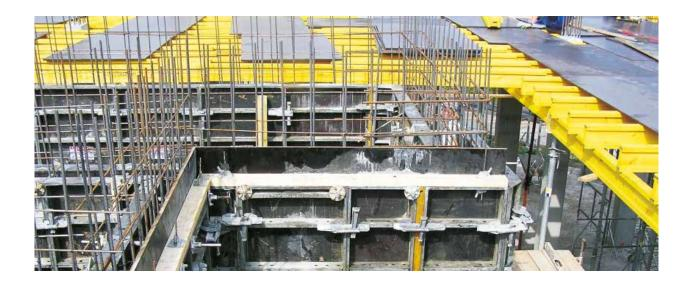
These system supports are made of steel hot dip galvanized pipes. The support height can be adjusted within 1,482 mm up to 5,500 mm. The wide adjustment range allows you to precisely compensate the ceiling surface and the ground irregularities.
