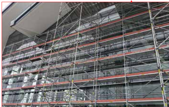
Works at the airport building facade
